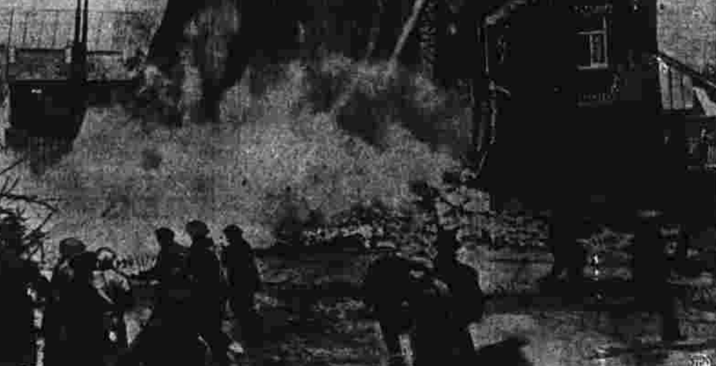
Camera's Eye Spots Disaster As It Happens In the remarkable photograph above, the camera caught the full tragedy of a disaster that left 200 Belgians of the village of Courcelles homeless, when a subterranean landslide caused buildings to collapse and roof tiles.
